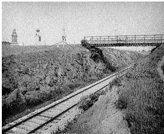
Railroad Cut just to the north of the Chambersburg Pike
